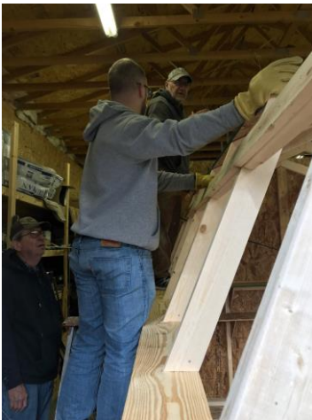
Knight Jacob Ridgway helps Habitat for Humanity build a new shed.
